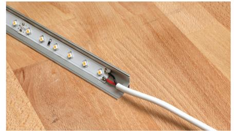
3. Insert the tape light into the channel by peeling off the cover on the adhesive backing and pressing the tape in a straight line from one end of the channel to the other to ensure flat, even adhesion.
